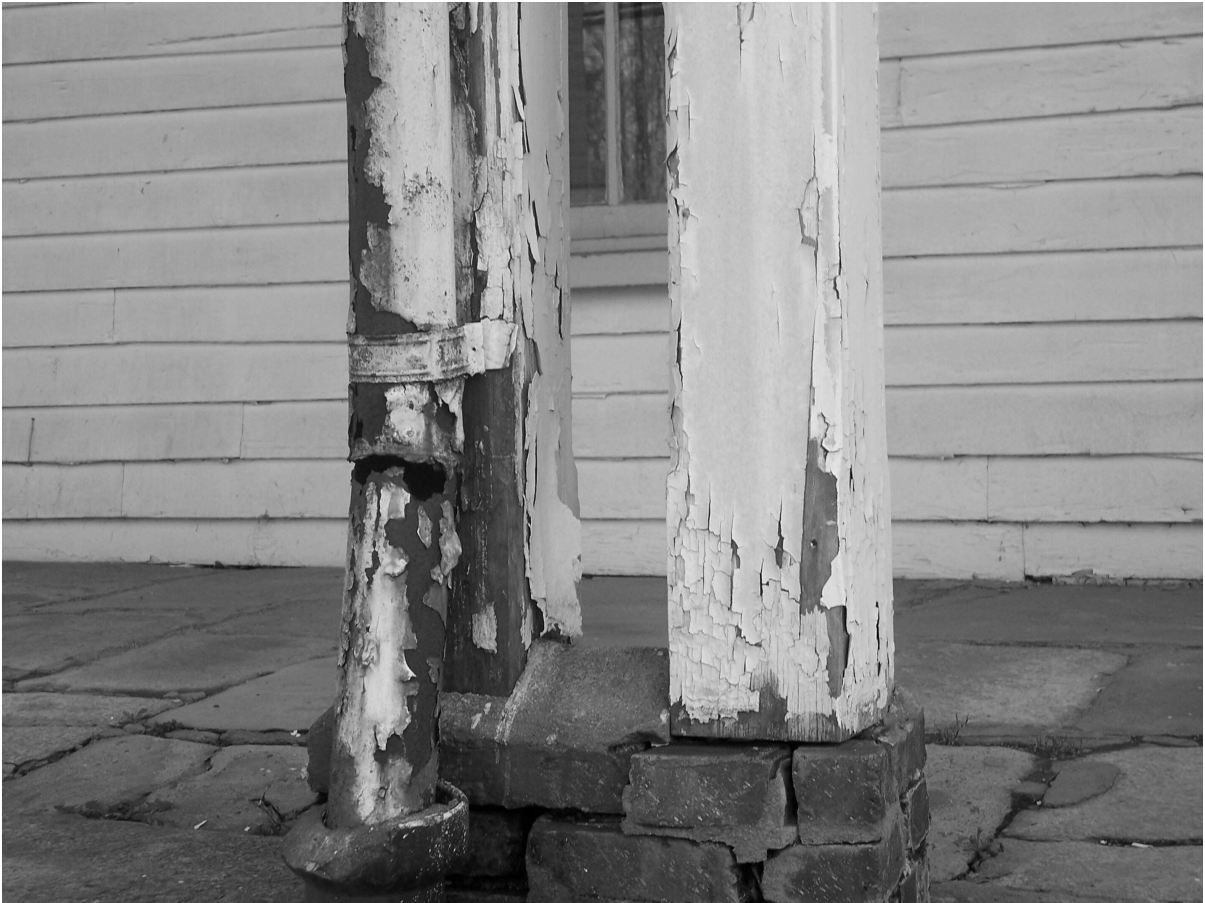
Figure 4: Colonial Inn, deterioration visible on the front porch. (Photo: Cheryl D. Warren, 2005)
